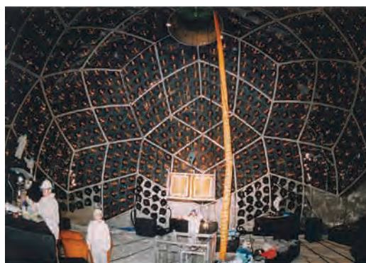
Inner view of KamLAND taken at the construction. Fifty centimeters diameter photo-sensors are installed inside the 18-m diameter sphere.
