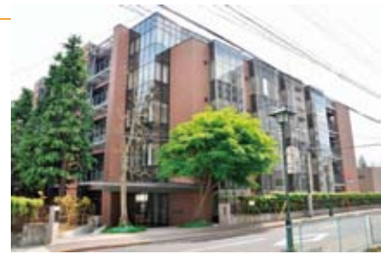
WPI Laboratory Building
