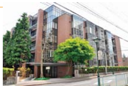
WPI Laboratory Building
