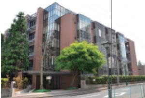
Appearance of the building
